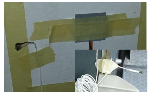
Figure 2: Above: Measurement set-up; heat flux sensor with inside temperature sensor, Bottom right: outside temperature sensor
