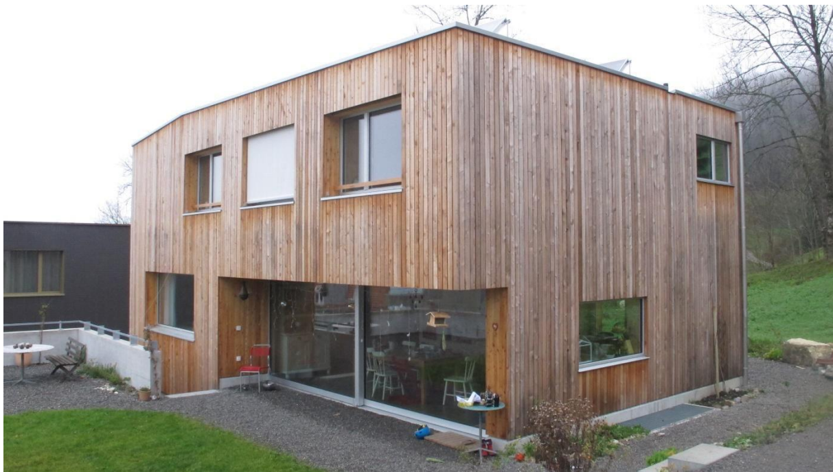
Figure 6: Swiss Minergie-certified building used for long-term measurement
